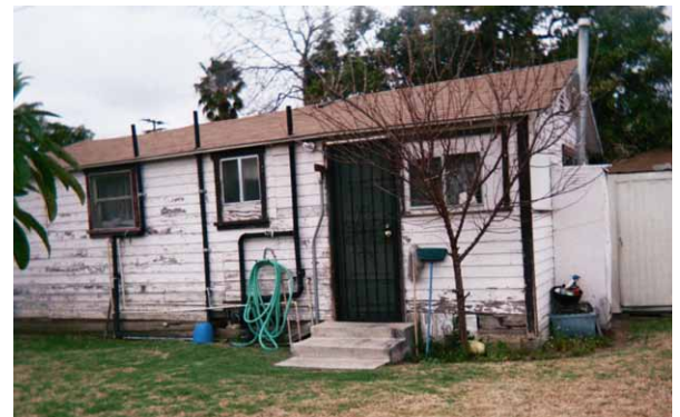
Existing farmworker housing in need of repair. Photo courtesy of Cabrillo Economic Development Corporation.
