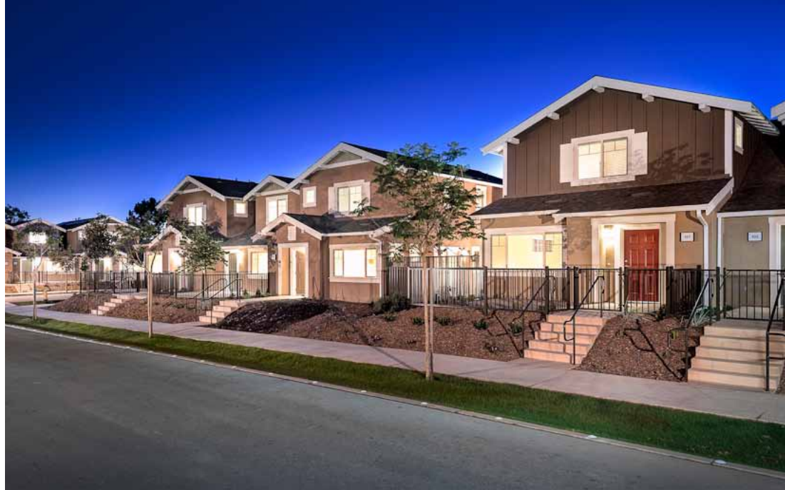
New farmworker housing in Ventura County. Photo courtesy of Stephen Schafer, Schaf Photo Architectural Photography.
