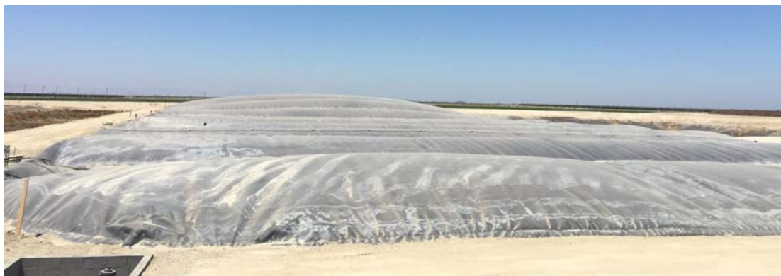
Image 5. Covered lagoon digester at Verwey-Madera Dairy.
