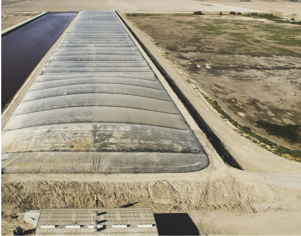
Image: Aerial view of the Verwey-Hanford Dairy Digester (Source: CDFA)
