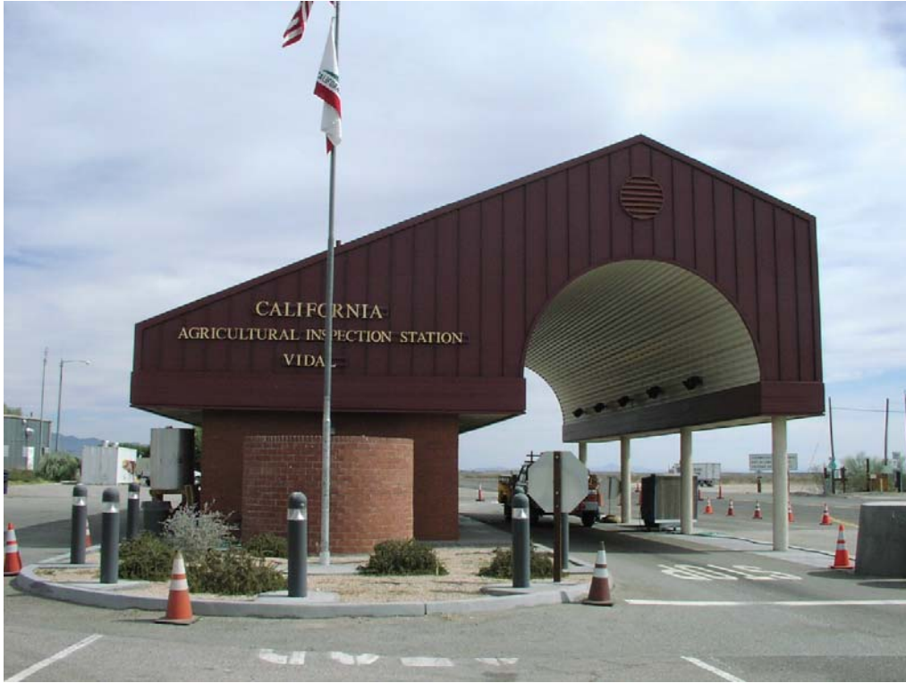
Vidal Junction Station
