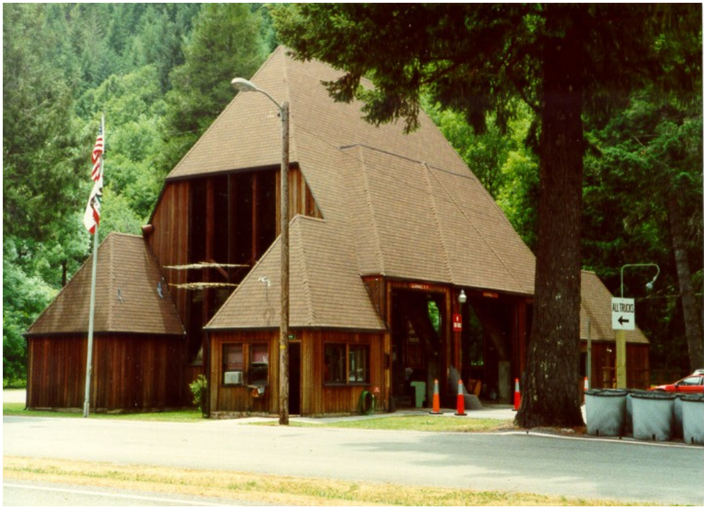
Redwood Highway Station
