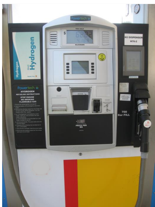
Photo 30: Hydrogen fuel dispenser
