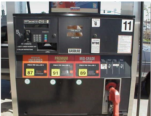
Photo 8: Multigrade fuel dispenser
